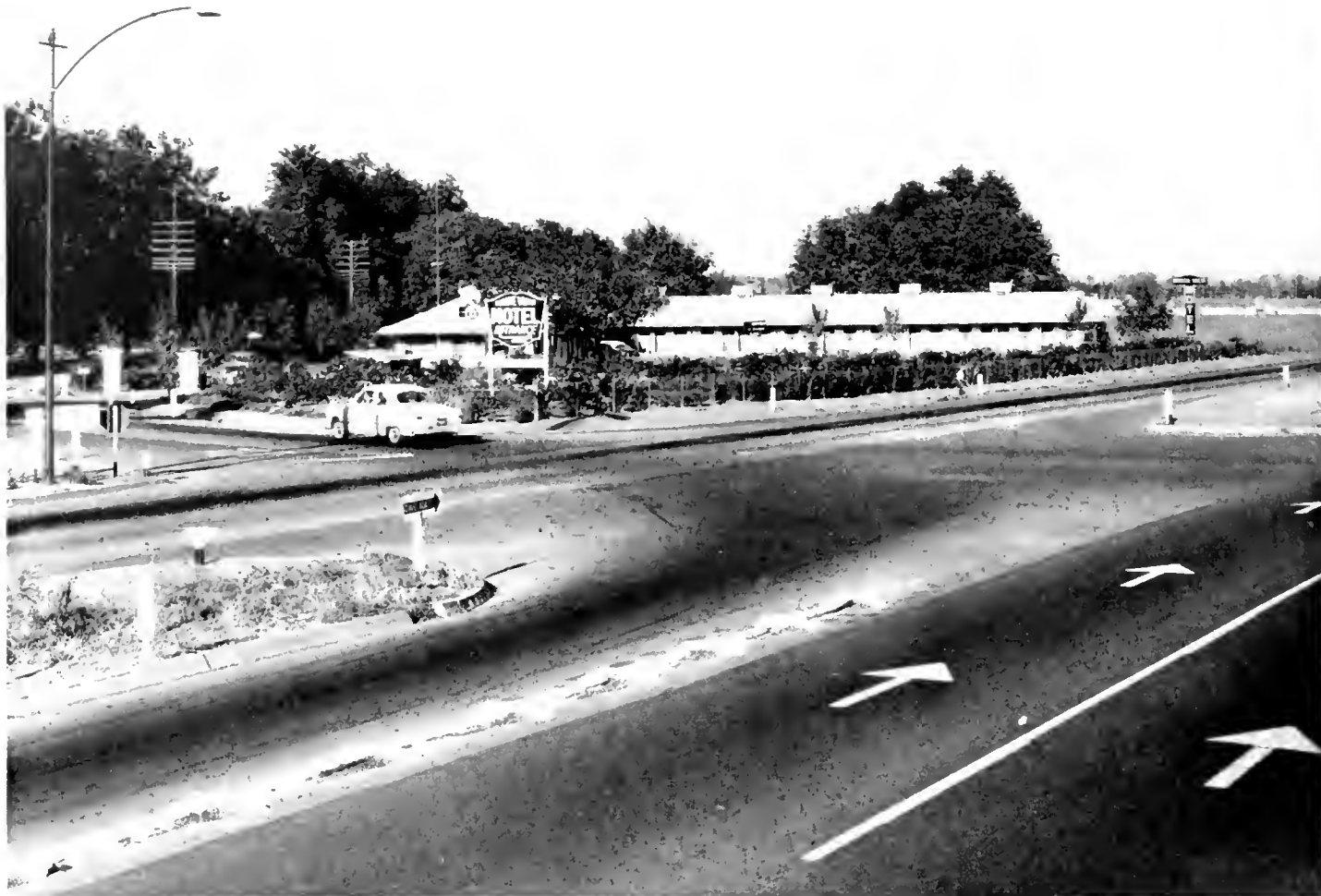
PHOTO 1—Motel on expressway near Vacaville. Access restriction along expressway requires motorists to drive on intersecting road to enter motel property. In the left portion of photo the entrance is identified by stone pillars.
